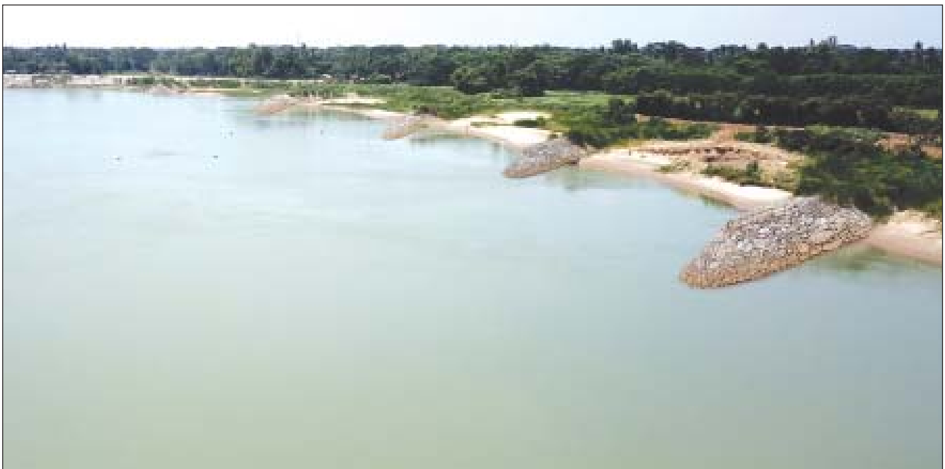
Repair & Restoration of Right bank of River Subarnrekha near village Rasalpur
