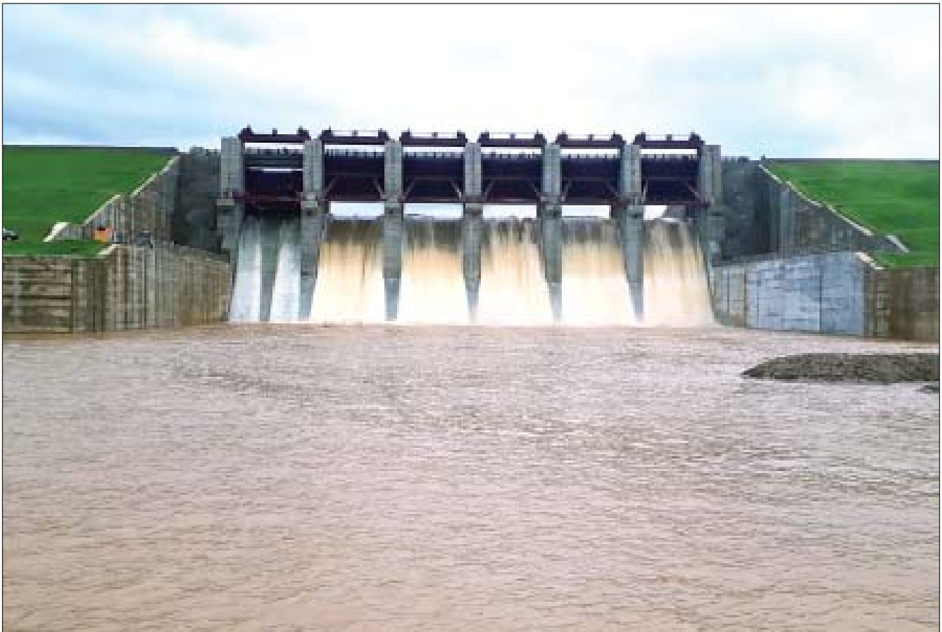
Ret Irrigation Project in Kalahandi Dis-
