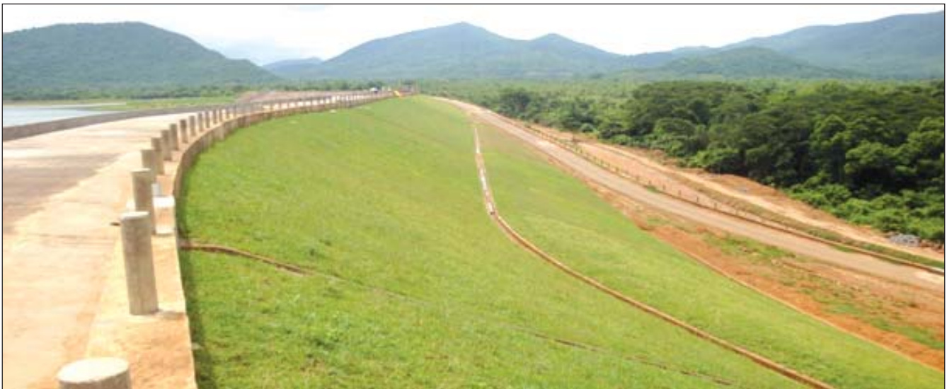
Down stream slope of Dhanei Dam after execution
