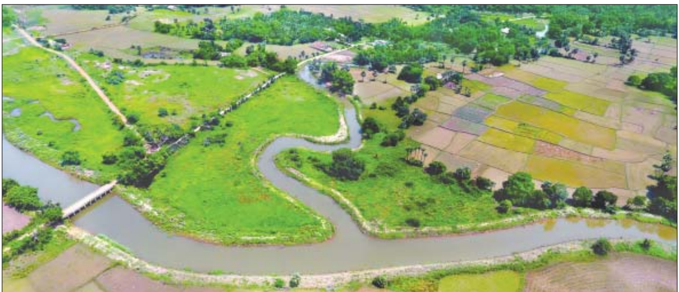
Improvement to Mantei Drainage Cum Creek with its right side link drains in Bhadrak District
