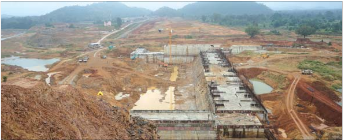
Lower Suktel Irrigation Project (Dam under construction) under WSIDP
