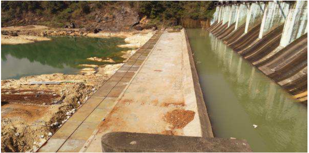
D/S APRON OF SPILLWAY
