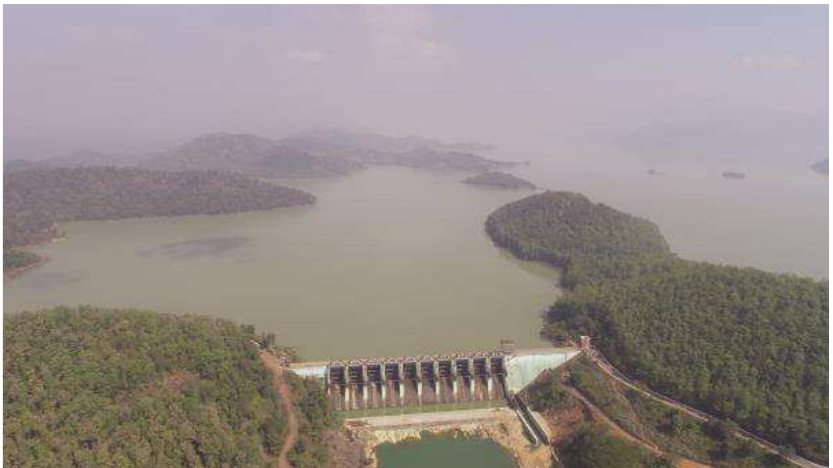
RESERVOIR AREA WITH SPILLWAY
