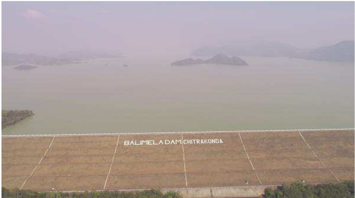
MAIN EARTH DAM
