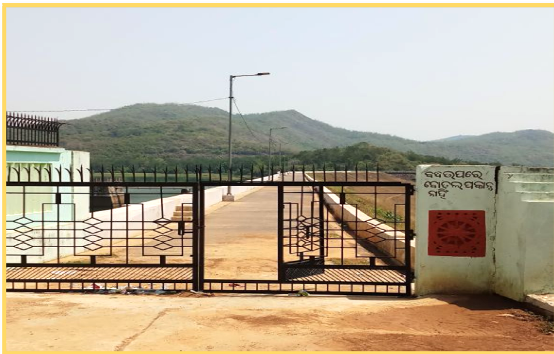
Salia Dam Gate
