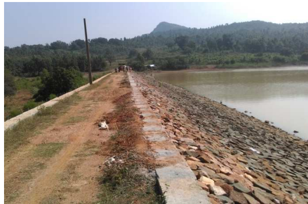
Repair of upstream slope riprap at Sanamachhakandana MIP under DRIP project
