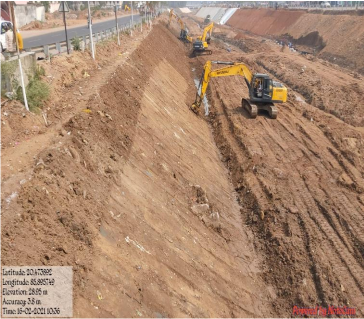
Profiling the Canal Section
