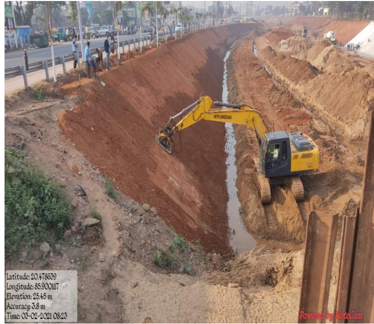
Compaction using moorum admixture
