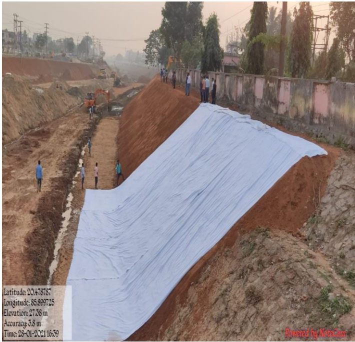
Laying of Geo-textile synthetic mattress
