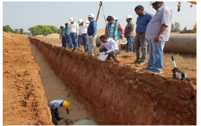
Sand bedding before GRP pipe laying
