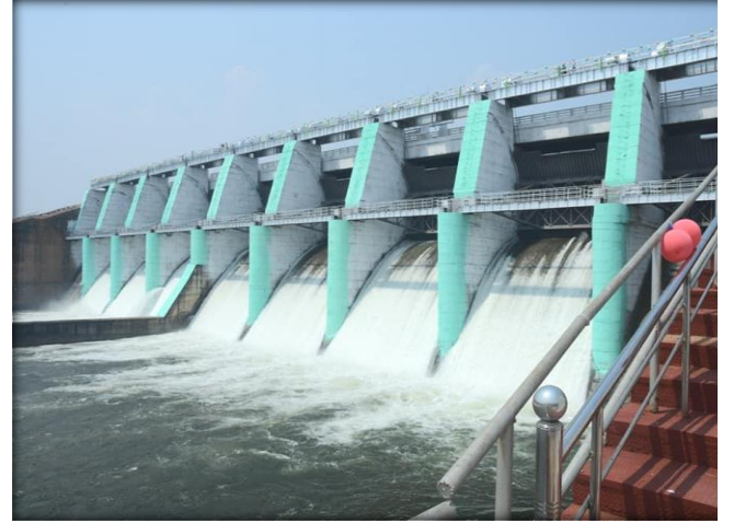
D/S view of Spillway
