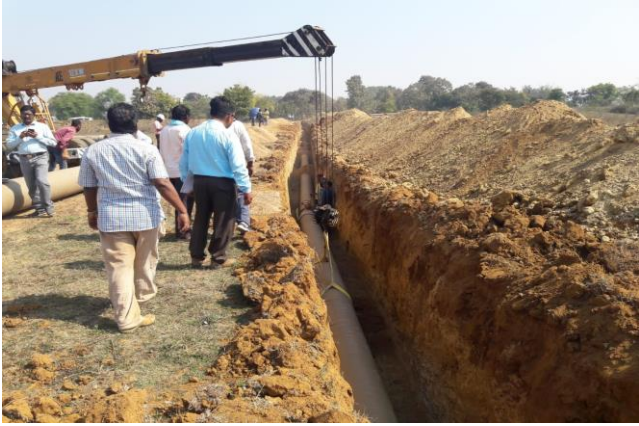
Laying of GRP pipe
